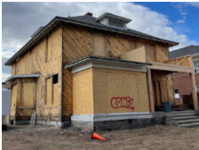
455 Hill Street today, under construction. Photo courtesy Debbie Hinman.
