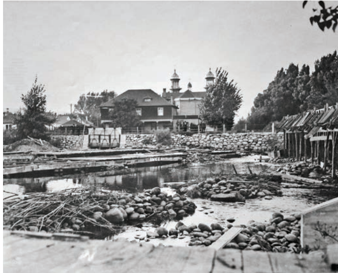
Construction of Arlington Bridge North, 1920. The Nevada Club is on the site of today’s 20th Century Club, and the spires of St. Thomas Aquinas are in the distance. Courtesy Neal Cobb.
