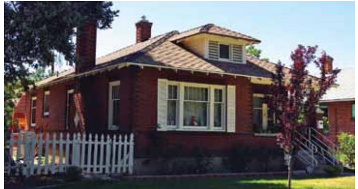
This Craftsman style cottage retains its original wood windows with divided upper lights, often referred to as "Craftsman windows."
