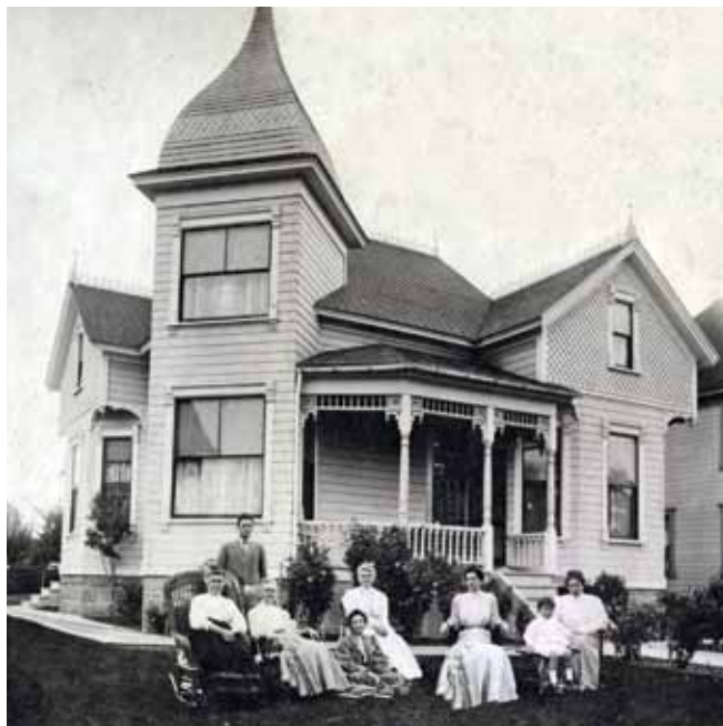
829 N. Center St., built c. 1895, demolished in 2020. Owned by the Folsom family until 1943, when it was purchased by the Atcheson family.
