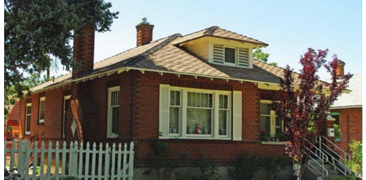
An example of a hipped dormer on a Craftsman cottage.
