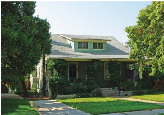
Shed dormer on a Craftsman style residence on Ridge Street.
