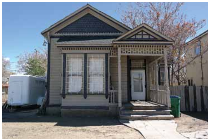
626 Center Street, a 19th century Folk Victorian style, built between 1885 and 1890.
