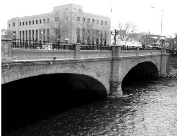
The Virginia Street Bridge at age 107, the 1934 Art Deco Post Office on the left and the 1926 Riverside on the right. Courtesy Kim Henrick.
